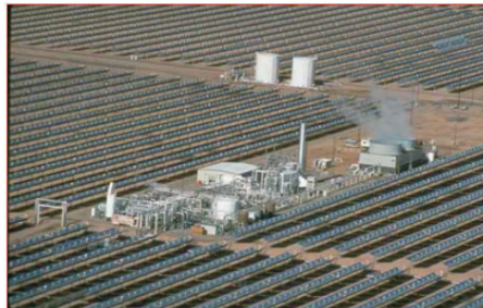
Commercial Trough System in California
