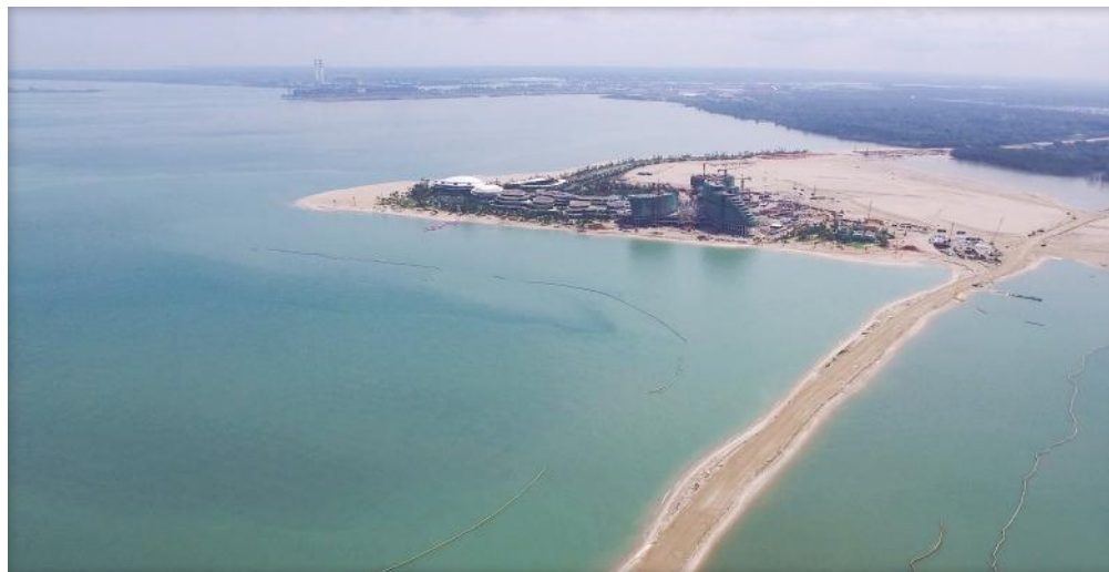
Figure 34 . An aerial view of the Forest City development on reclaimed land, Johor Bahru. Photo Credit: Marcel Williams, 2017.
